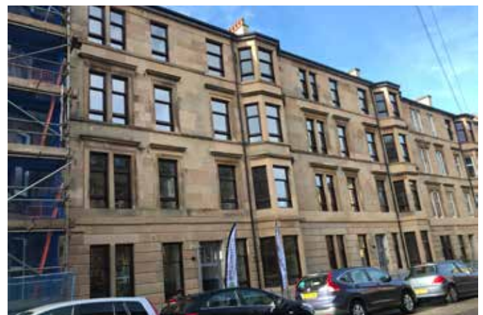
Improved flats at Annette Street
