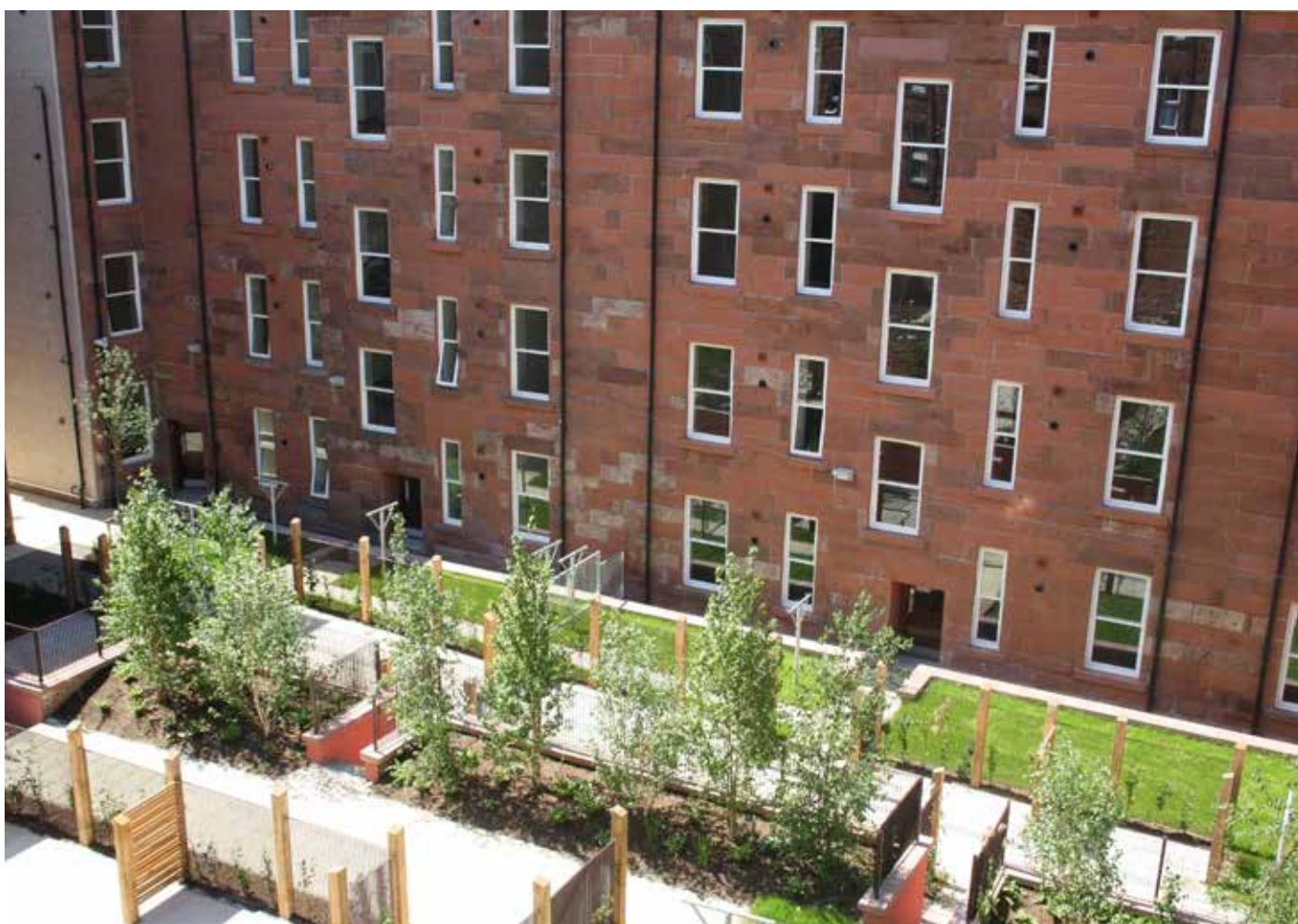
Backcourt before and after Ancroft Street/ Nansen Street, Queens Cross Housing Association
